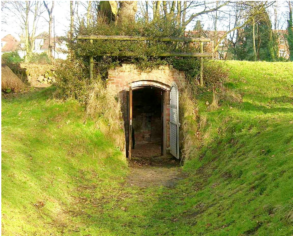
Figure 13: The icehouse in Moseley Park.
