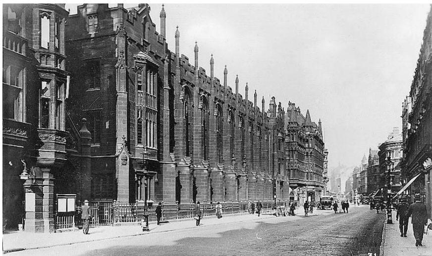
Figure 43: King Edward's School, New Street, Birmingham.
