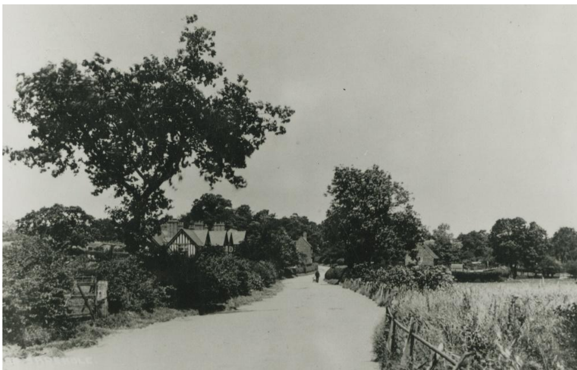
Figure 37: The gables and chimneys of Gracewell Cottages from the south.
